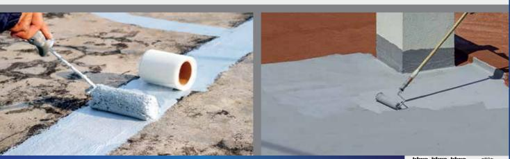
COLD POLYUREA is a two component, fast curing, cold applied polyurea waterproofing membrane. It creates an elastic and durable film layer on the surfaces. PU 650 TC-1K or PU 600 TC-1K should be used as a top coat in order to use it in places exposed to UV and outdoor effects.
