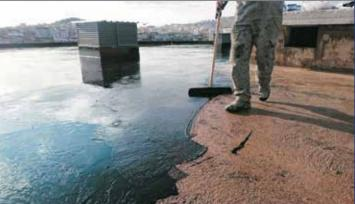
PU 650 2K AQUA is a two-component, polyurethane based, 100 % aliphatic top coat membrane. Especially in swimming pools, applying on epoxy or polyurethane coating products, creates a protective coating that is UV resistant and chlorine resistant.
