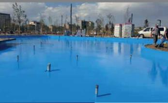
SLC 1100 is a single component, 100% silicone based, highly adhesive, solvent-free, UV resistant, flexible waterproofing membrane curing with the humidity in the air.
